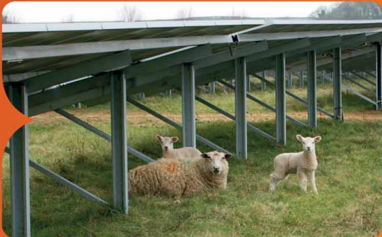
Solar PV modules mounted onto arrays
