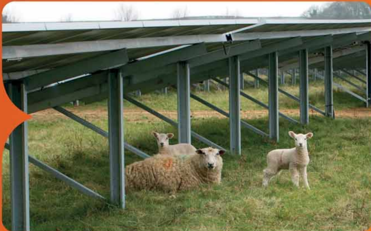
Solar PV modules mounted onto arrays
