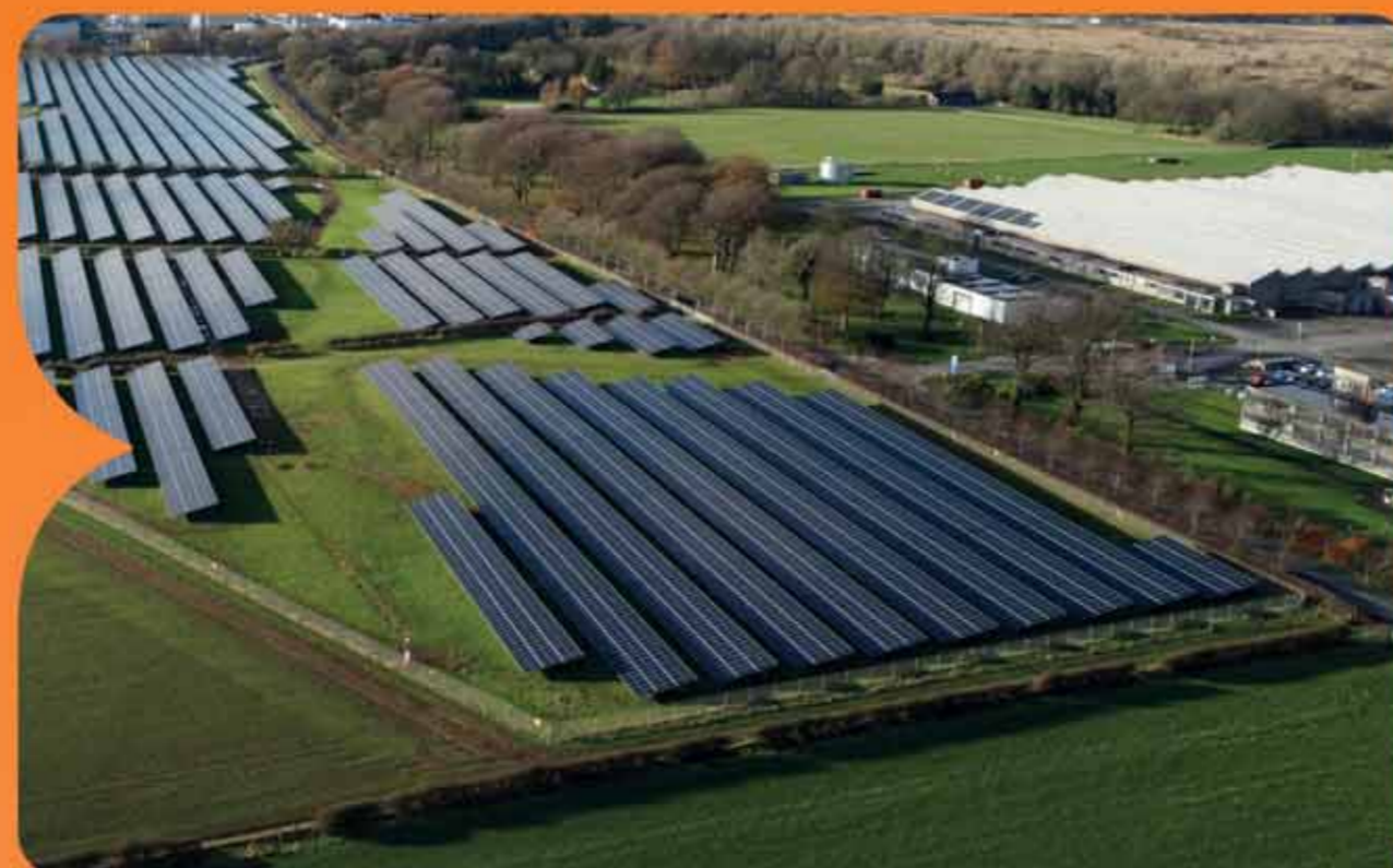
Access tracks and landscaping in and around the site
